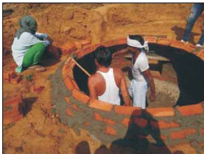
Plastering of digester wall during CMC
