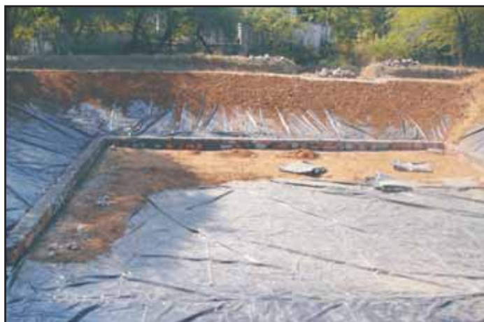
LDPE lined Farm pond for Rain water harvesting (under construction)
