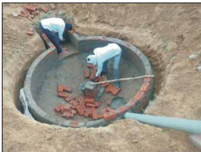
Construction of digester wall during CMC
